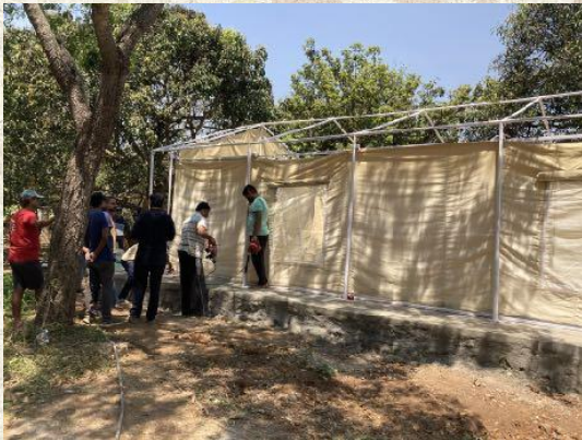
Mounting the tent fabric on to the framework
